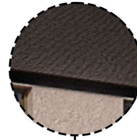
ROOF SLATE AND OFF-WHITE RENDER
